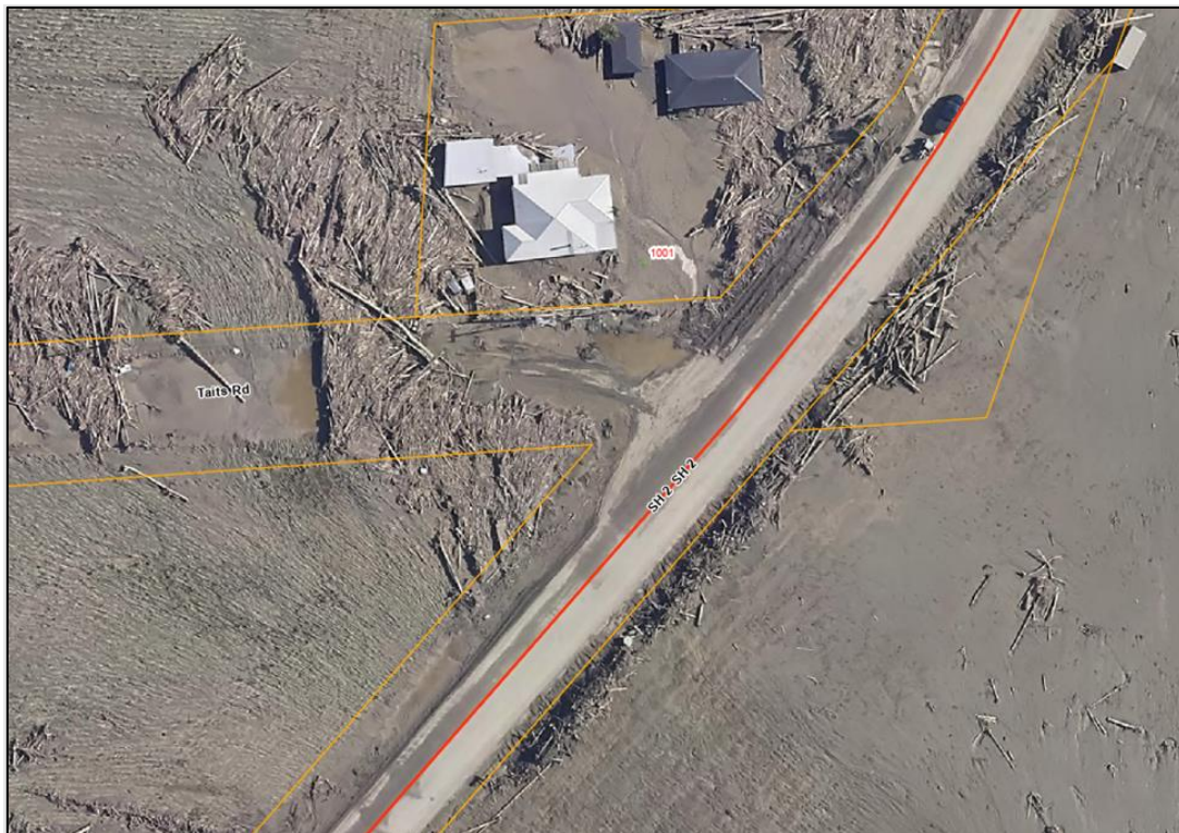
Figure 13.1 - Woody Debris build-up near Esk River mouth.
