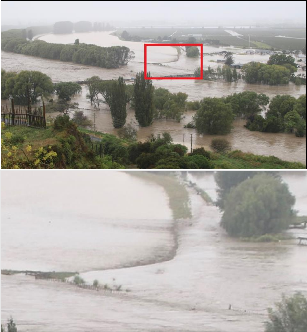
Figure 40.3 – Photos showing water flowing back into the Tutaekuri river at the approximate location of the designated breach site
